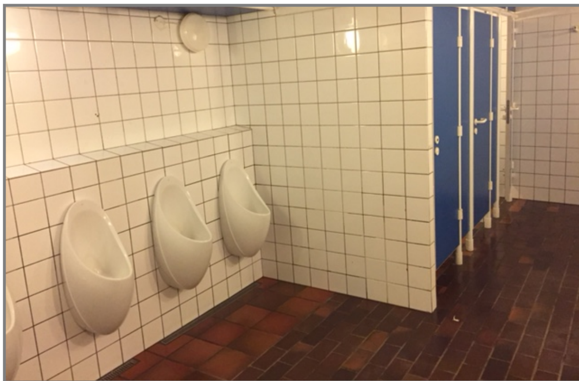
A toilet in a school is now fresh and odor-free thanks to treatment with Prebona DuraClean and Prebona OdorControl.
